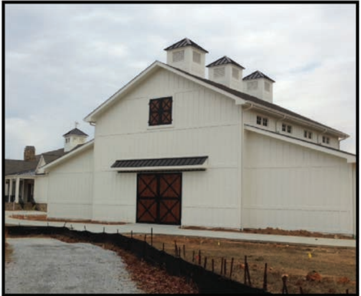
Solid Wood Fill Sliding Barn End Doors with Cross Bucks & Hinged Loft Doors with Cross Bucks
