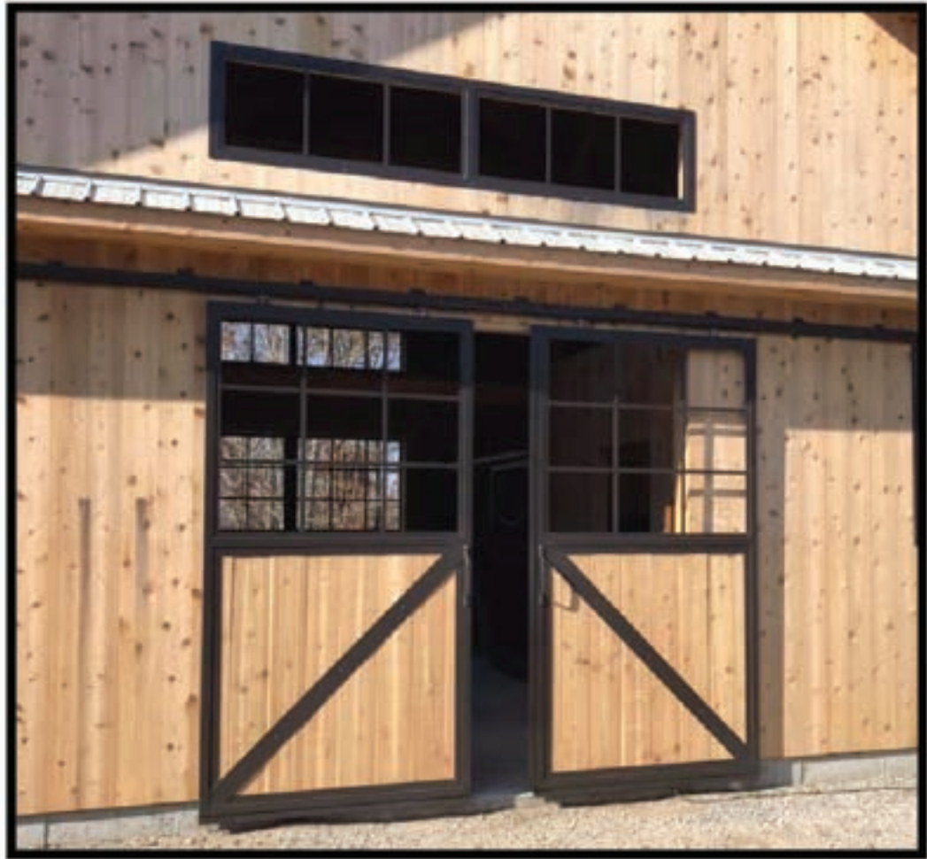
Glass Topped Barn End Door with Welded Cross Members & Vertical Wood Fill with Transom
